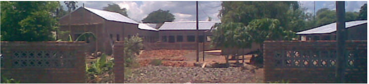
The Kuwangisana community centre buildings in Sena are nearing completion!
